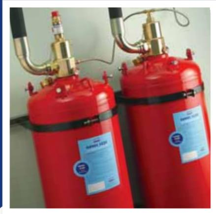
**NOVEC 1230** is supplied in lightweight cylinders with a small footprint that requires minimal storage space. Novec 1230 fluid has a boiling point of 49 degrees C and therefore exists as a liquid at room temperature. It is super-pressurised with nitrogen to 25 bar and rapidly
