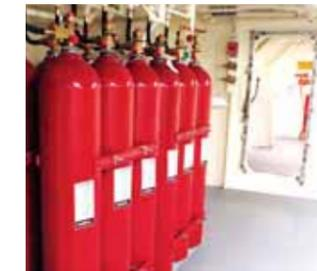
It expands at a ratio of 450 to 1 by volume. For fire suppression purposes, the discharge is designed to displace the air containing oxygen, which supports combustion, and results in fire extinguishment.
